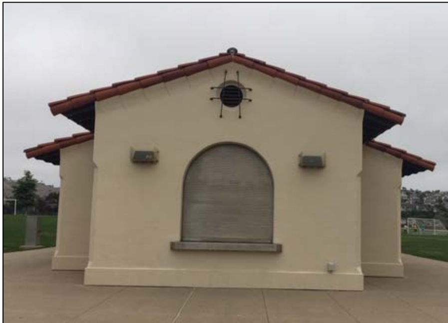
Example of an Ancillary Municipal Snack building with the slaking of the stucco at the edge of the tile roof.
