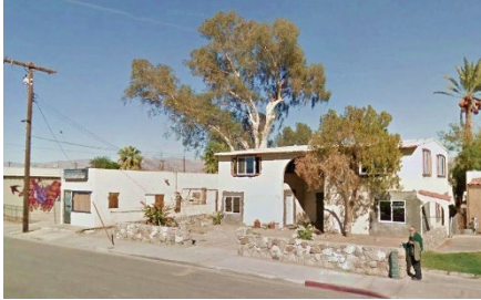
Existing Buildings. SOURCE: Michael Baker International
