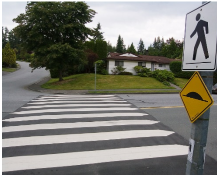
Raised Crosswalk. SOURCE: Richard Drdul
