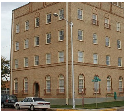
Rectangular and Arched Windows, Double Hung Windows and Framing. SOURCE: Jeffrey Beall
