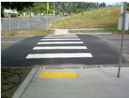
Raised Crosswalk. SOURCE: Scott Batson
